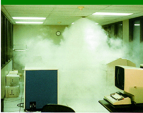
FM200 GAS DISPERSION INSIDE DATA CENTER.
